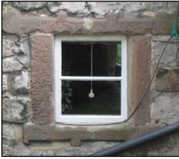
P34 Townhead House – re-used lintel and cill
