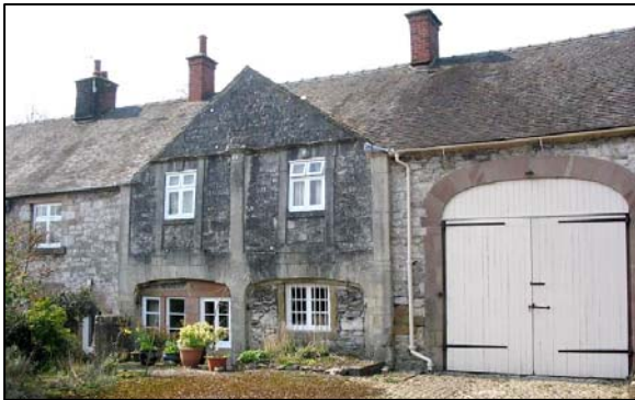
P38 Stabling to south of the Hall
