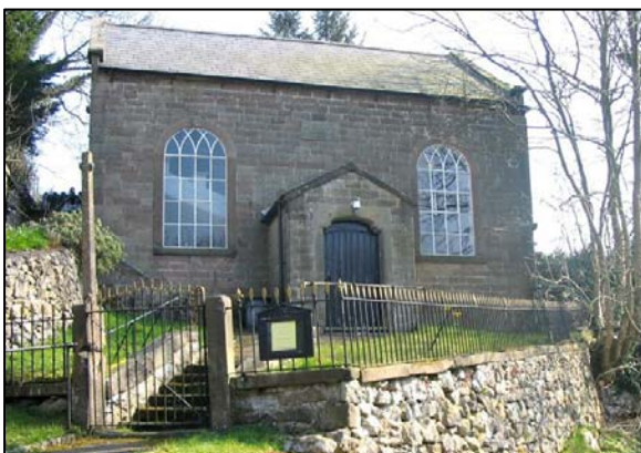
P48 Parwich Methodist Church
