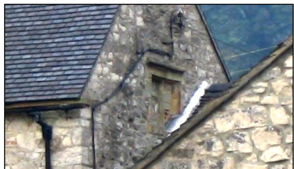
P33 Nethergreen Farm - blocked C17th window
