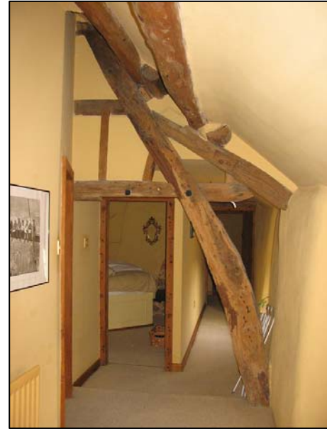
P37 Cruck beams inside Shaw Lane House
