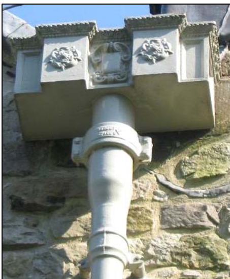
P52 Cast iron rainwater goods
