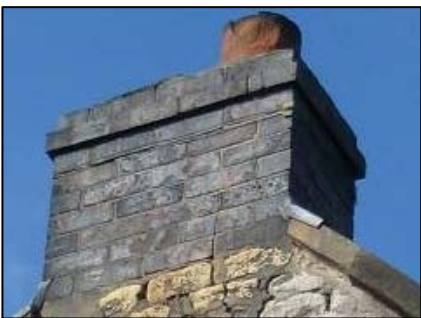
P63 Engineering blue brick chimney stack
