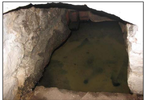
P46 Well in basement at Fernlea
