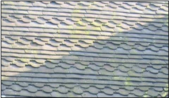
P62 Fishscale clay roof tiles
