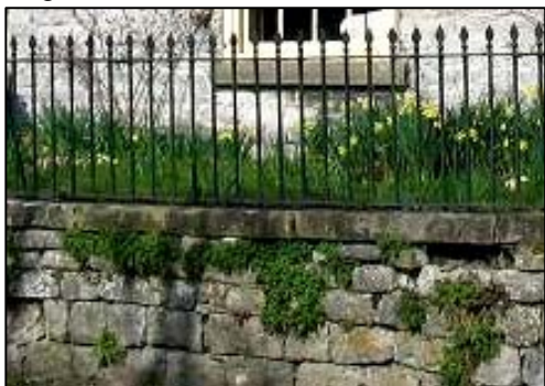
P56 Decorative iron railings at Sunnside
