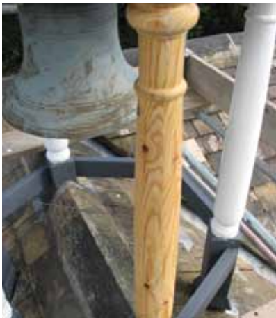
Grant-aided repairs to the bell tower at Hassop Hall Stables
