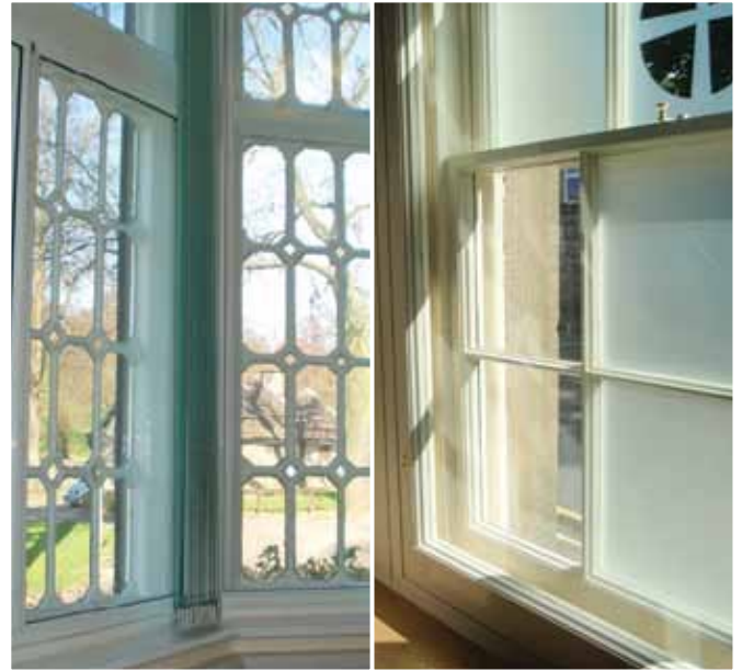
Secondary glazing to a traditional single-glazed window
