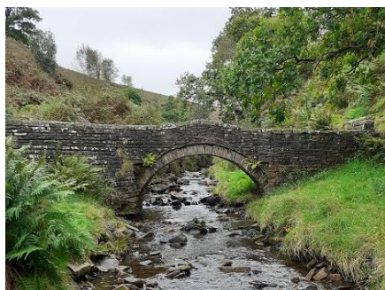
Historical Packhorse Bridge by River Goyt Upstream Site
