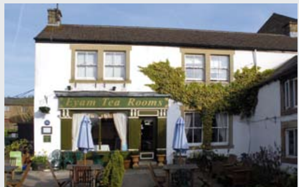
After: openings reduced in width; more traditional windows and shopfront surround added
