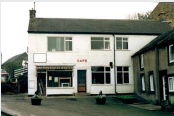
Before: showing inappropriate openings and details
