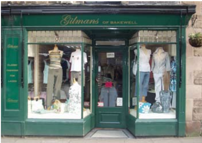
Traditional shopfront Bakewell
