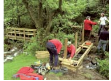
National Park maintenance team replacing footbridge at Highlow
