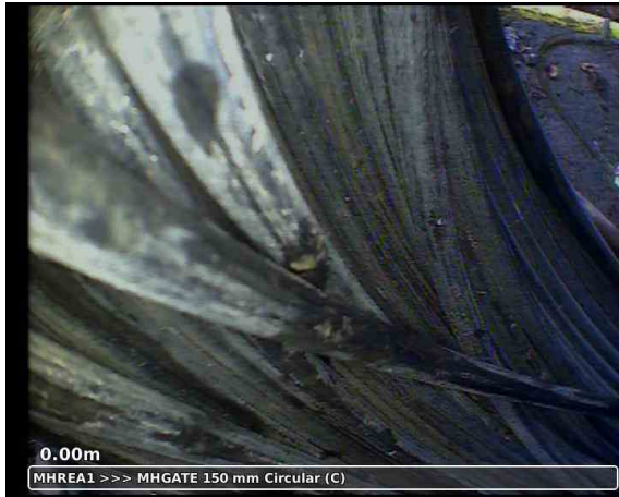
20240212-000011-snap0000.jpg, 00:00:05, 0.00 m Start node, manhole, reference: MHREA1
