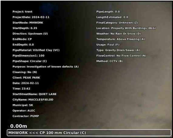
20240211-234448-snap0000.jpg, 00:00:02, 0.00 m Start node, manhole, reference: MHWORK
