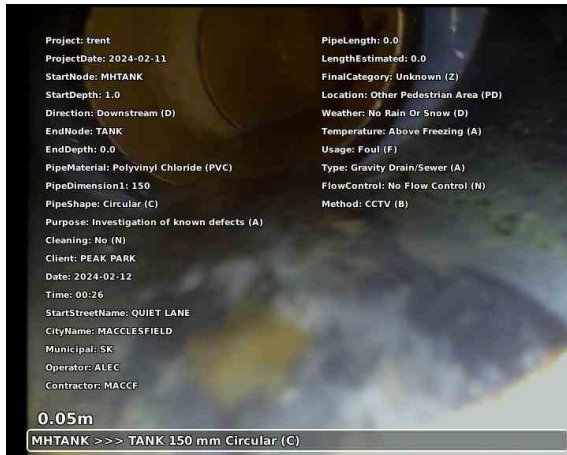
20240212-002705-snap0000.jpg, 00:00:02, 0.00 m Start node, manhole, reference: MHTANK
