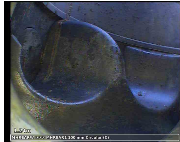
20240211-235501-snap0001.jpg, 00:00:18, 1.24 m Finish node, manhole, reference: MHREAR1
