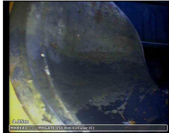
20240212-000011-snap0001.jpg, 00:00:36, 4.05 m Finish node, manhole, reference: MHGATE
