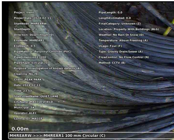
20240211-235501-snap0000.jpg, 00:00:02, 0.00 m Start node, manhole, reference: MHREARW
