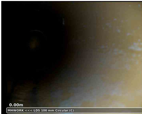
20240211-234549-snap0000.jpg, 00:00:05, 0.00 m Start node, manhole, reference: MHWORX
