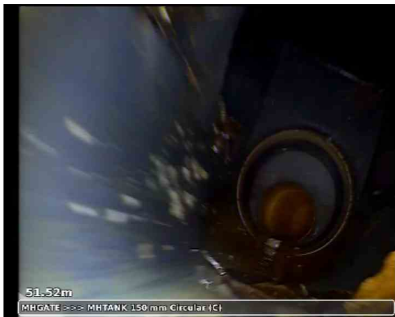
MHGATEX_425fbec7-be0a-4570-bd14-0eac48b2df77_20240216_144748_534.jpg, 00:00:09, 51.52 m Finish node, manhole, reference: MHTANK
