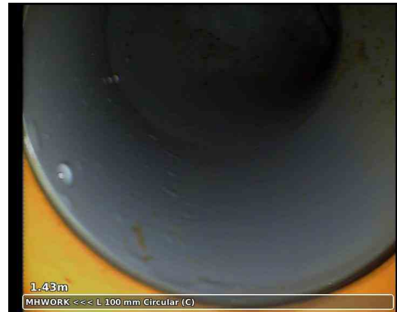
20240211-234716-snap0001.jpg, 00:00:16, 1.43 m Survey abandoned, Rest Bend Ladies
