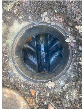
MH Rear 1 - Internal
