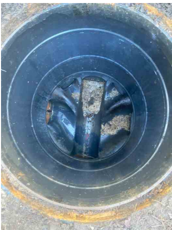
MH Gate - Internal
