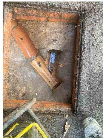
MH Rear Workshop - Internal
