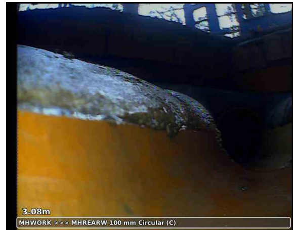
20240211-235009-snap0001.jpg, 00:00:28, 3.08 m Finish node, manhole, reference: MHREARW
