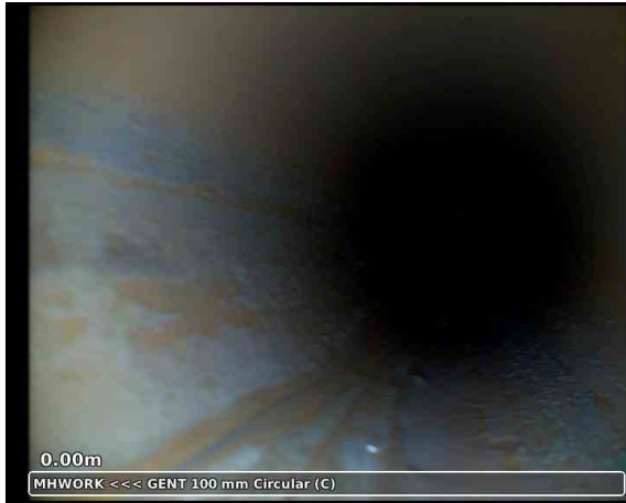
20240211-234826-snap0000.jpg, 00:00:03, 0.00 m Start node, manhole, reference: MHWORX
