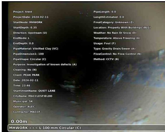
20240211-234716-snap0000.jpg, 00:00:02, 0.00 m Start node, manhole, reference: MHWOK
