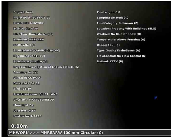
20240211-235009-snap0000.jpg, 00:00:02, 0.00 m Start node, manhole, reference: MHWORX
