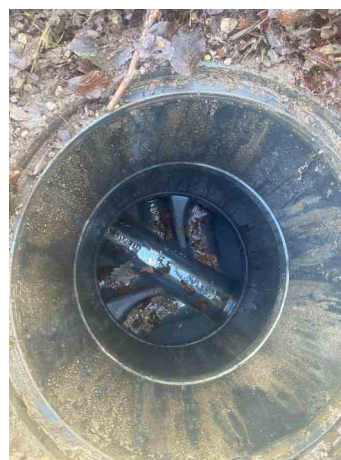
MH Septic Tank - Internal
