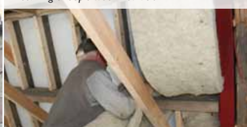
Installing sheep's wool insulation
