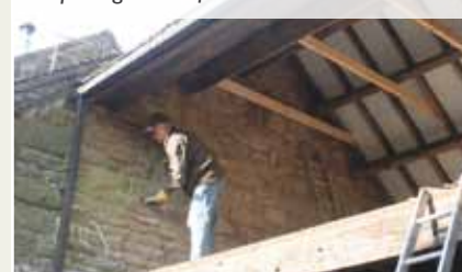
Preparing a wall for lime mortar
