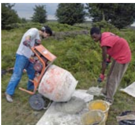
Volunteers mix special plant-friendly cement to restore a 100-year-old wall on Ramsley Moor, near the Sheffield border.
