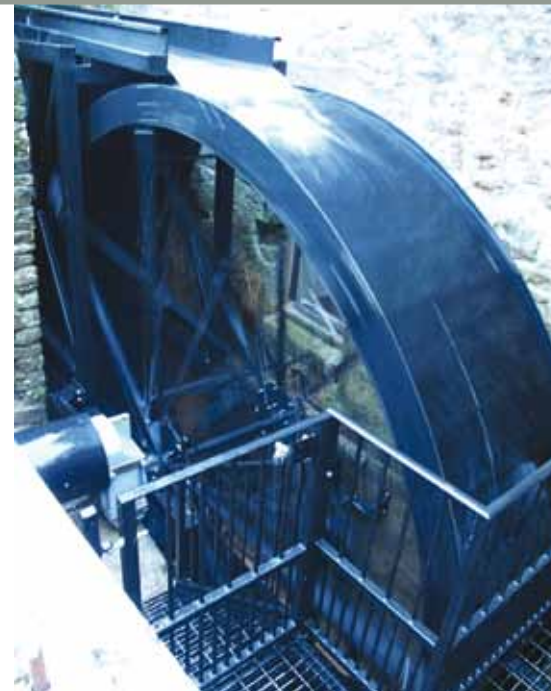
Above: A 4kW capacity waterwheel in a micro-hydro electric scheme at a house in Calver. The converted corn mill was one of the sites highlighted in Friends of the Peak District's Peak Power report. © Graham Woods, Friends of the Peak District.
