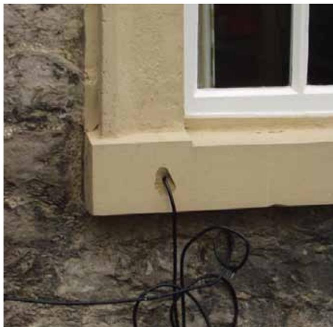
*This picture shows the effect of a poorly sited cable and the damage done to an historic window, by insensitive drilling*
